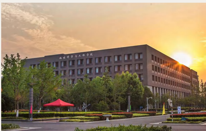
School of Earth Sciences and Engineering Nanjing University Xianlin Camups
